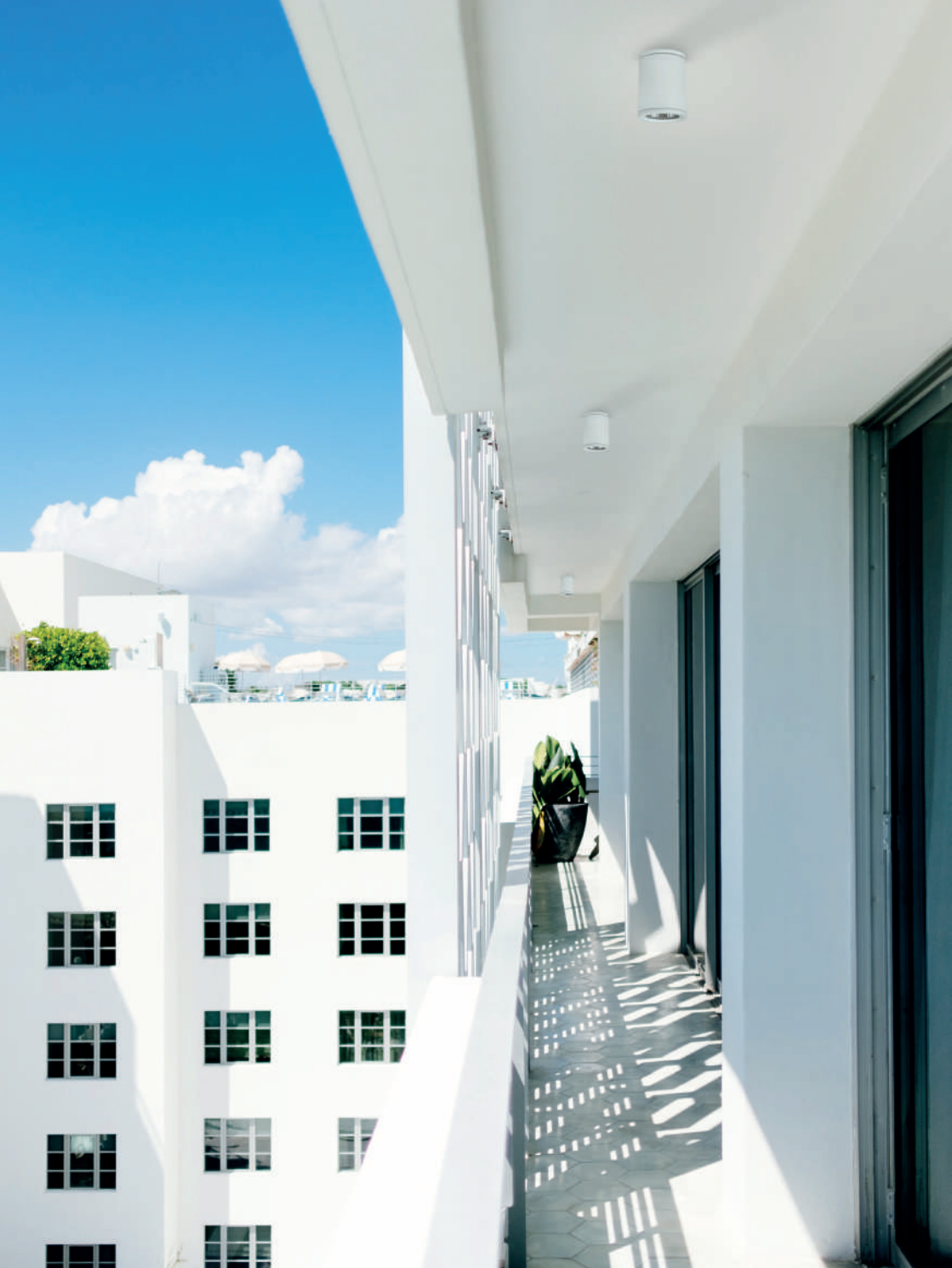
OUTDOOR - CEILING FIXTURES
