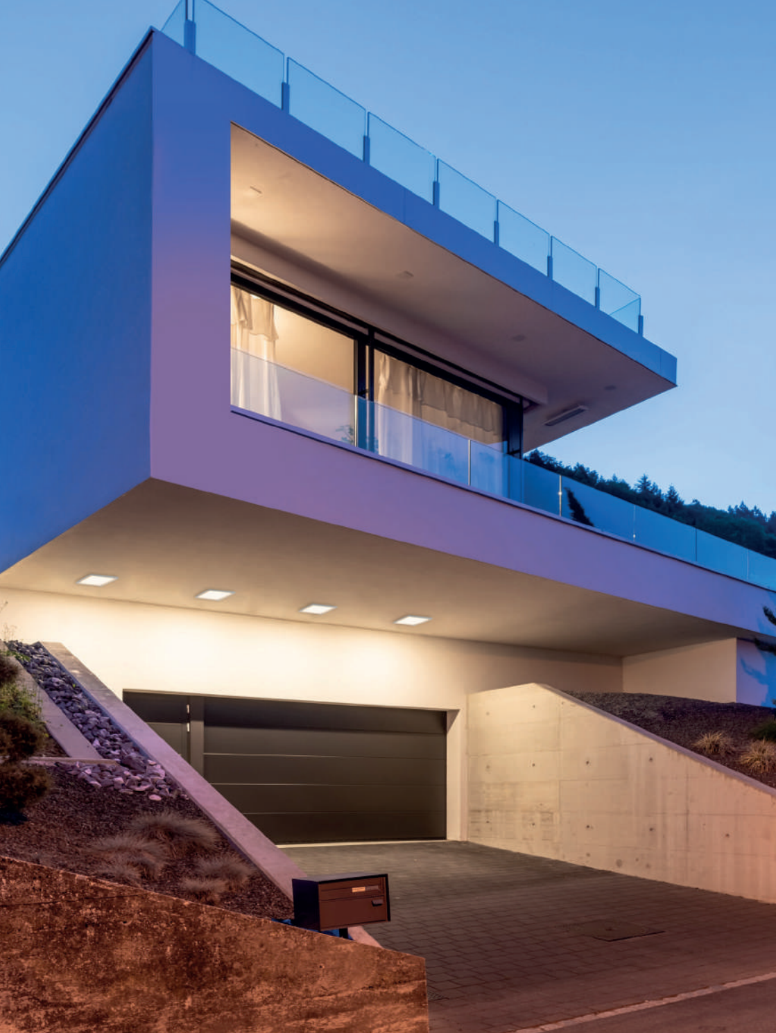
OUTDOOR - CEILING FIXTURES
